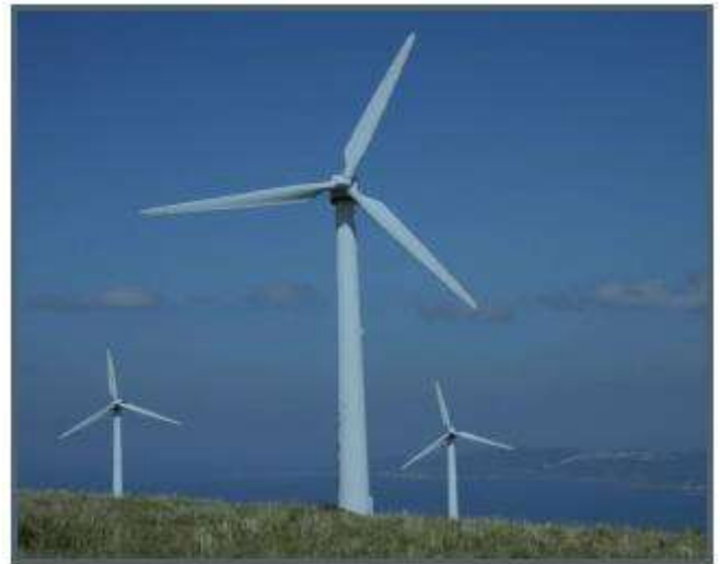
Fig.2. NEG Micon 1.5MW Wind Turbine, 68m diameter Rotor, Tubular Steel Tower. Blades are made up of fiberglass. The Rotor blades can be Turned to optimize power & the entire tower is rotated to face the wind. Most breeze turbines begin creating power at twist speeds in the request of 3-4 meters for each second (m/s) (8 miles for every hour); produce an "ostensible" greatest power at around 15 m/s (30 mph); and close to stop the harm of the
